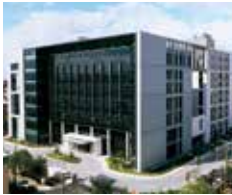
Taoyuan Technology Center (Green Building)
